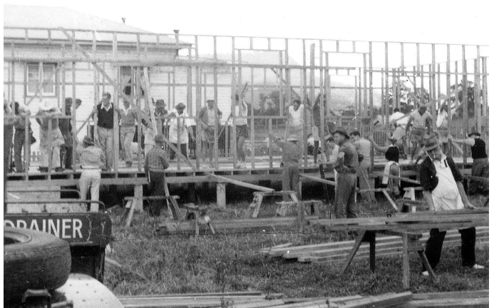
The stud walls are up! (photo courtesy of Quentin Snow)
