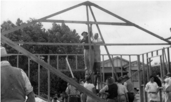
The first roof truss goes up (photo courtesy of Quentin Snow)
